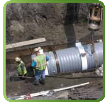
Sliplining and Trenchless Applications
