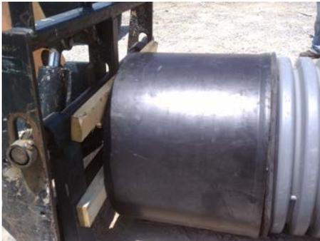
Be sure to lube both gaskets and the leading edge of the adapter. It is important not to damage the adapter during the installation. Additional end protection such as 2x4's or a wooden skid may be necessary to install the adapter. With construction equipment, push the adapter over the end of the pipe that will be installed in the MH.
