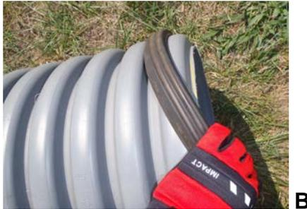
Carefully begin to position the gasket on to the pipe and “roll” it to the 4<sup>th</sup> corrugation valley, figure B, C, D, & E. A flat head screwdriver may be needed to aid in rolling the gasket down the pipe. Figure F shows the final orientation of the gasket with the lettering facing towards the end of the pipe and the gasket ribs firmly filling the corrugation valley.
