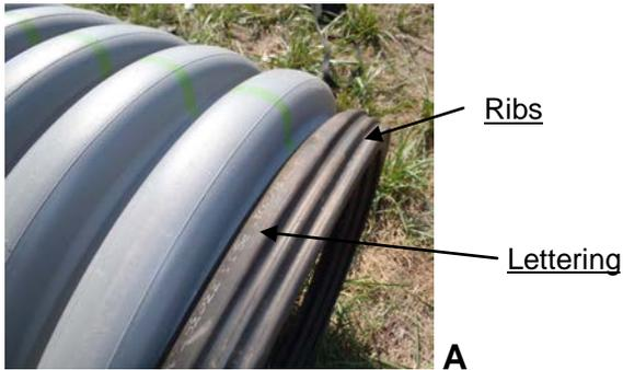
Depending on how the gasket arrives, one may need to twist the gasket so that the lettering is facing “out” and the ribs are furthest away from the pipe, figure A. Please note that this is the opposite way one would want to install the front gasket.
