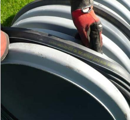
Place the front gasket into the first valley corrugations as shown to the left. The lettering will face the direction in which the adapter will be installed and the gasket will fully fill the valley corrugation.
