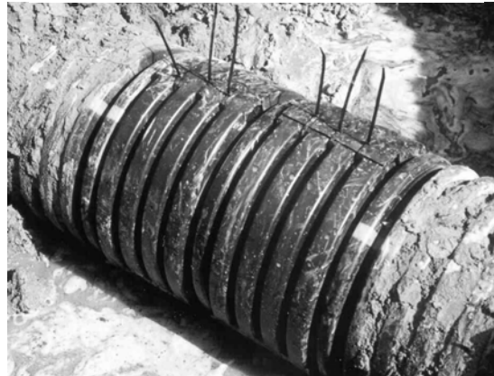
Figure 3 Split Band Installation
