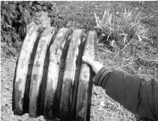
Figure 2 Pipe Cut Location
