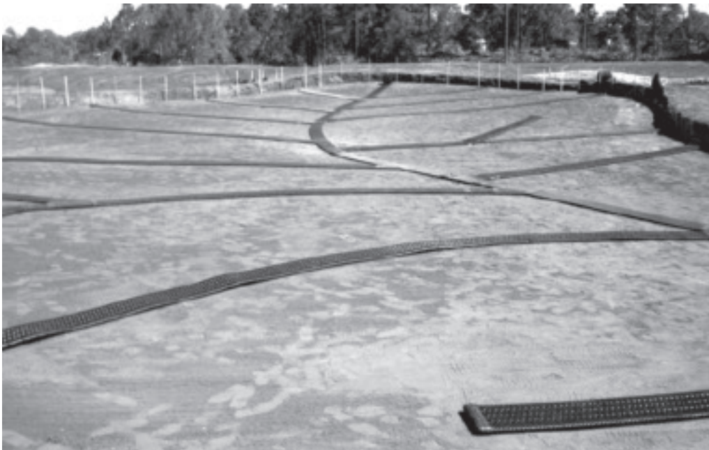
Figure 3: Typical green detail showing layout pattern incorporating AdvanEdge® fittings.
