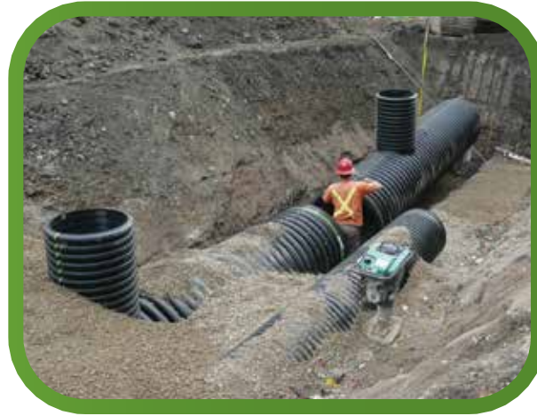
The ADS Water Quality Unit (above) is lightweight and easy to install, requiring little in the way of manpower or heavy equipment.
